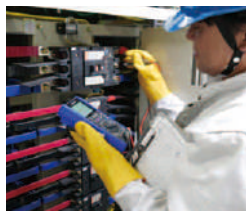
Secure the instrument on the wall so that you don't have to hold it.
